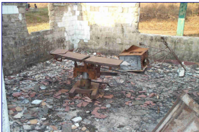
Burnt operating table in derelict Kambia Hospital
